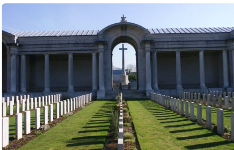
Buried/remembered at Arras Memorial (Bay 6), Pas de Calais, France
